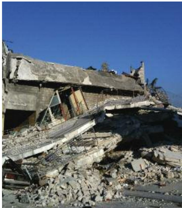
A HAITIAN NURSING SCHOOL REDUCED TO RUBBLE.
